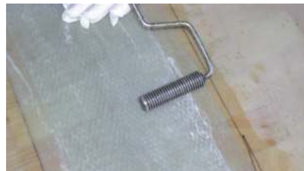
When you see fibres out of line(see above), drag your hand along behind it as you roll back.
